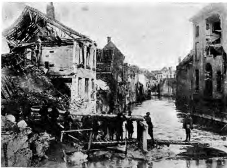
Placing abutment for bridge over canal in town of Audenarde. City was badly damaged by shell fire.
